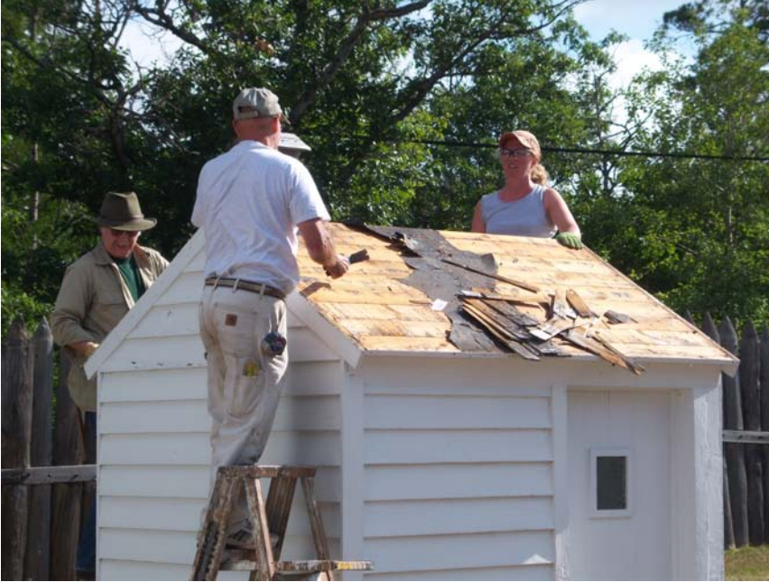
(Photo of Teacher Restoration Corps working on Privy roof)
